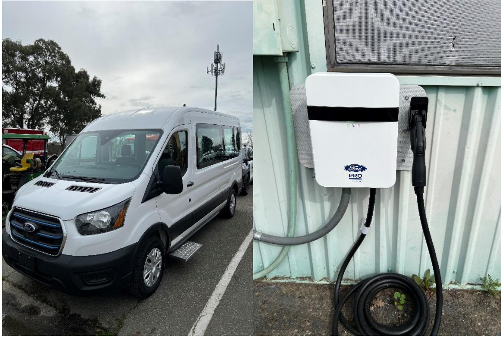
Fig 1. and Fig 2. The City of Davis' new electric van and charger, March 2024
